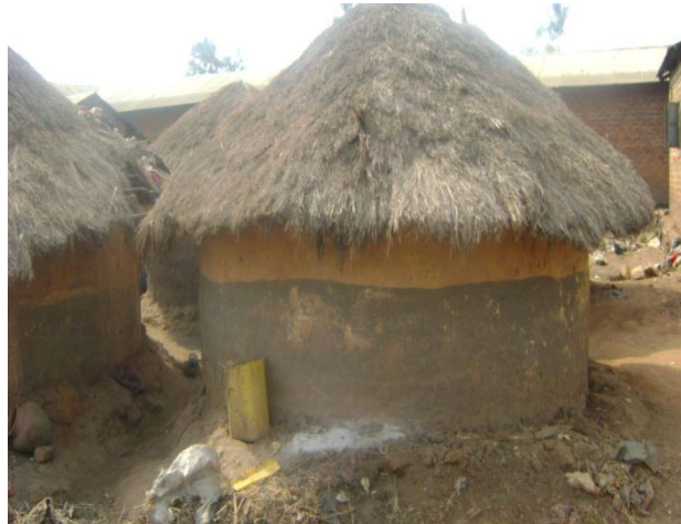
PLATE 1: A TYPICAL HOUSE FOUND IN MVULE (KIKARAMOJA)
